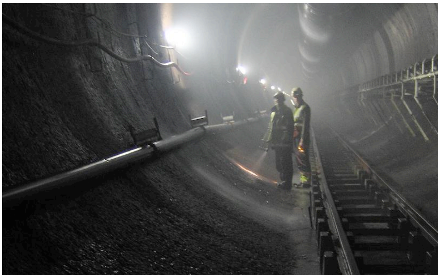
Figure 7. Photo showing tunnel inspections in TBM rear zone
